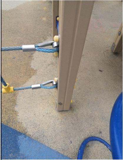
A close-up photograph showing the blue rope net fully secured to the metal post. The rope is wrapped around the post and held in place by a metal hook and a yellow plastic cap.       |
