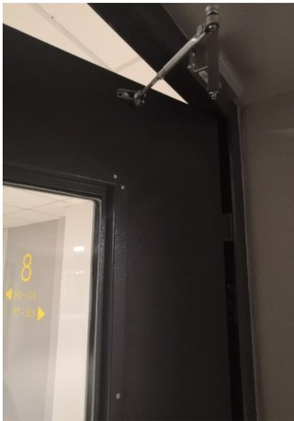
A photograph of the same door after the door closer has been secured. The door is now closed, and a yellow sign with the number "8" and arrows is visible on the glass part of the door. |
